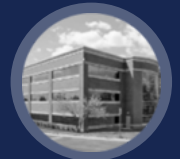
EXELON ENERGY PARK
